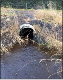
Figure 10.–Steam 4 sliplined culvert under Egan Drive.
