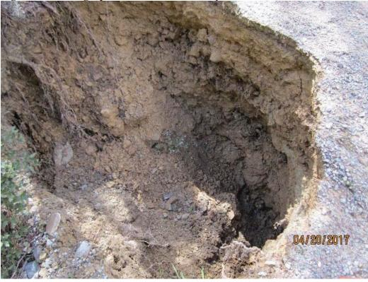
Figure 4A. Photograph of sinkhole created by failed culvert
