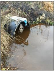
Figure 4.–Stream 1 sliplined culvert under Egan Drive.
