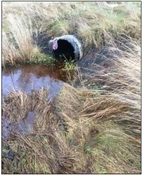
Figure 6.–Steam 2 sliplined culvert under Egan Drive.
