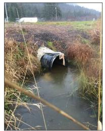
Figure 17.–Stream 7 sliplined culvert under Egan Drive.
