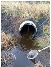
Figure 12.–Stream 5 sliplined culvert under Egan Drive.
