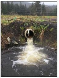
Figure 14.–Stream 6 sliplined culvert under Egan Drive.
