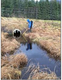
Figure 8.–Stream 3 sliplined culvert under Egan Drive.
